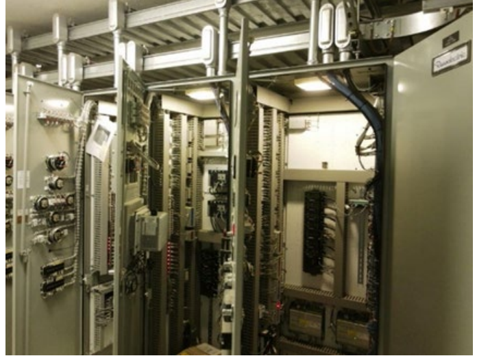
View of Control panels. The control room is equipped with the necessary panels for four generators
